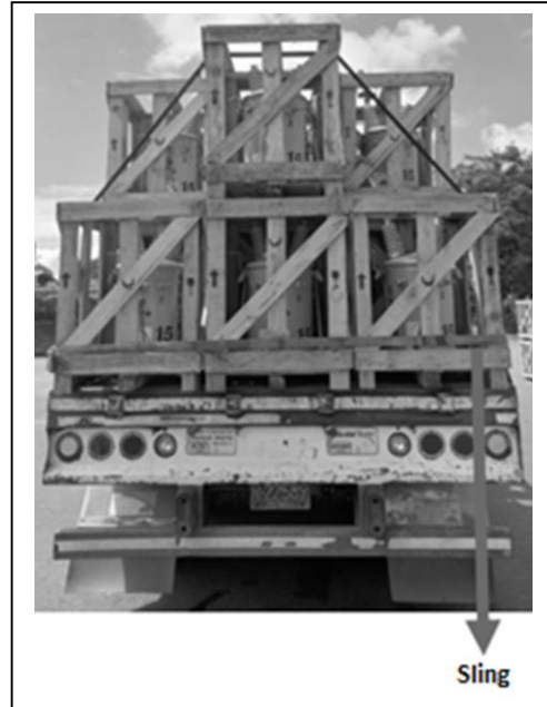
Figure 19: Securing the last row of loaded transformers
