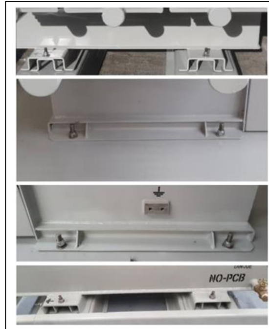
Figure 15: Anchoring the transformer to the base with screws
