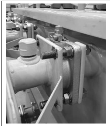
Figure 39: Loosen and remove nuts
