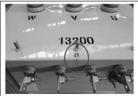
Figure 46: Security Seal
