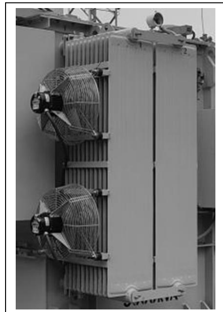
Figure 76: Installation of fans
