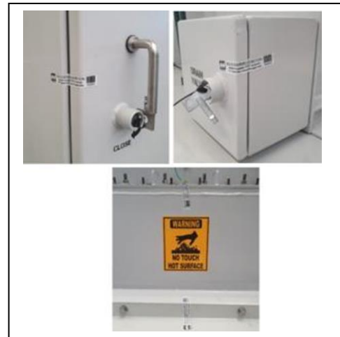
Figure 29: Security seal on removable parts
