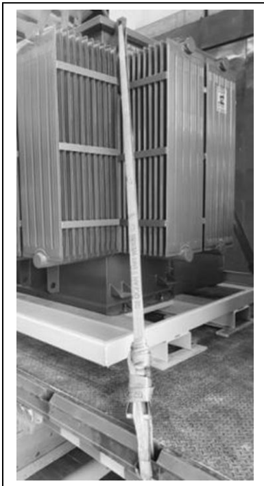
Figure 16: Example to secure the product with slings
