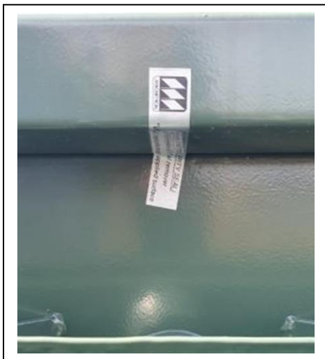
Figure 28: Seal of security cover-tank
