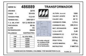
Figure 32: Example rating plate
