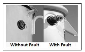
Figure 38: IFD in operation
